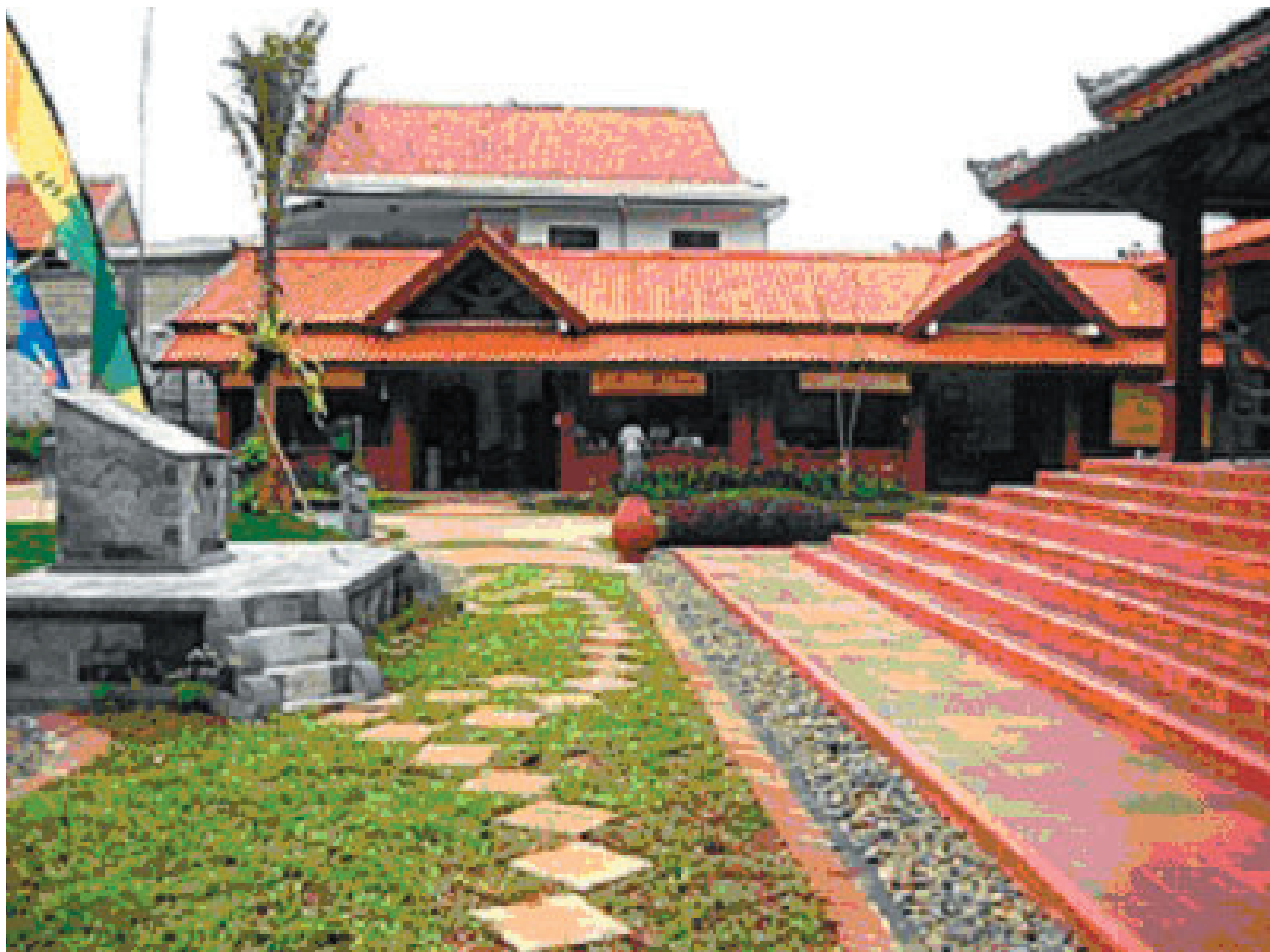
Entrance to the kite compound (top), with an appropriately symbolic pattern of bricks. Below, the store and workshop.
