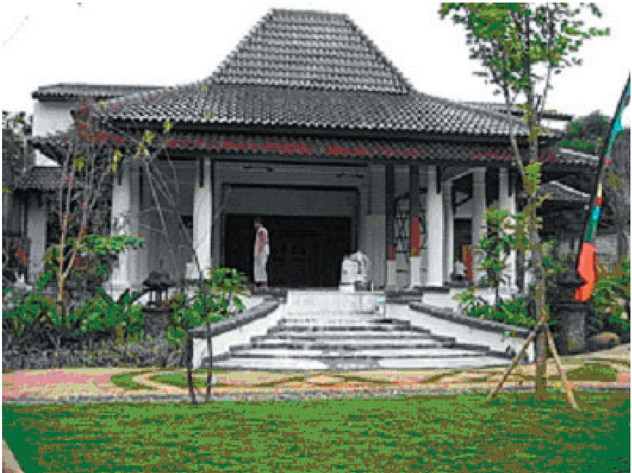
Top, the gazebo, a former Balinese rice barn. Below, a multipurpose building consisting of residence, guest quarters and extra workshop space.
