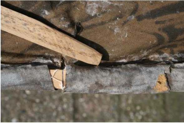
End of middle spreader is tapered
