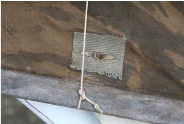
One of the two vertical tension lines fixed on one of the wing spars
